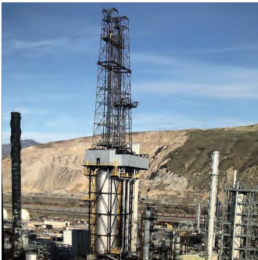
Figure 1 Two drum coker unit
